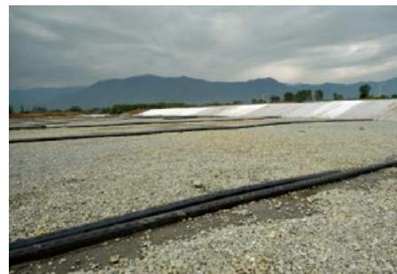
The underground drainage system for leachate collection
